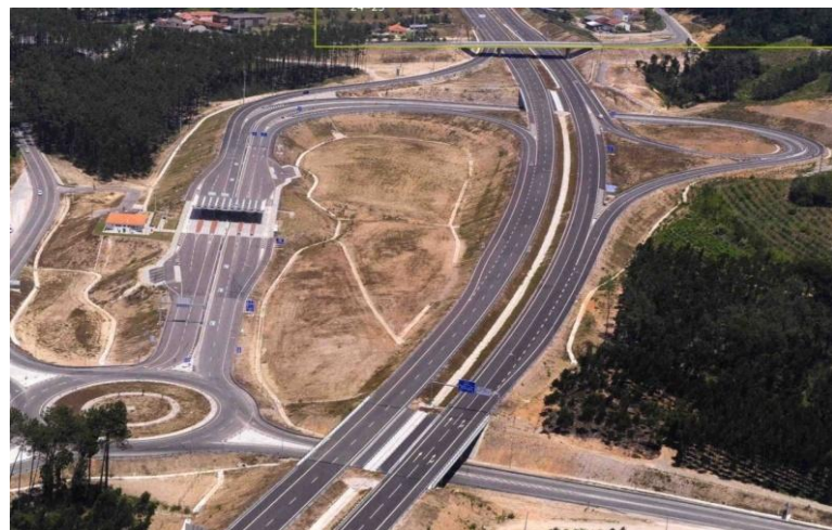
Road Junction (Leiria Norte)
