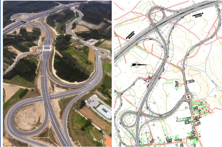
Toll Plaza in the Lourçal Road Junction
