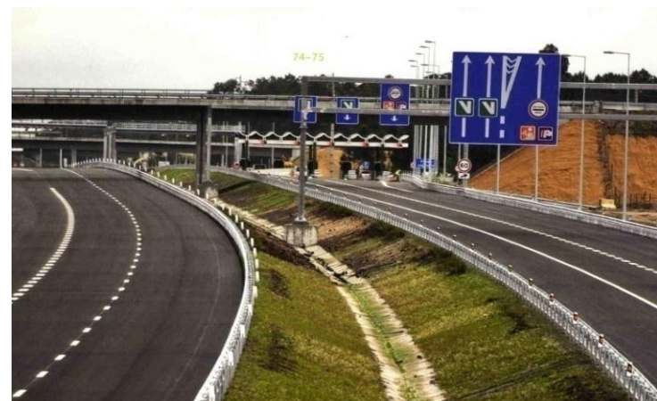
Toll Plaza in Current Section
