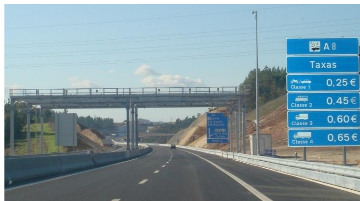
IC36 - Free Flow Structure
