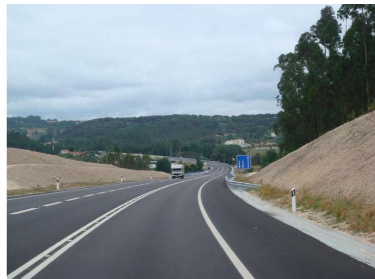
Overview of IC9/EN356 Road Junction
